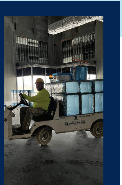
Dylan Gilbert staging materials for the job
